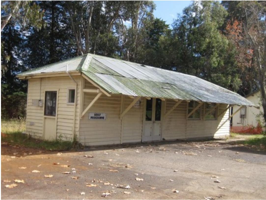
Figure 6.0 The 1936 shelter shed. (Source: GML 2012)
