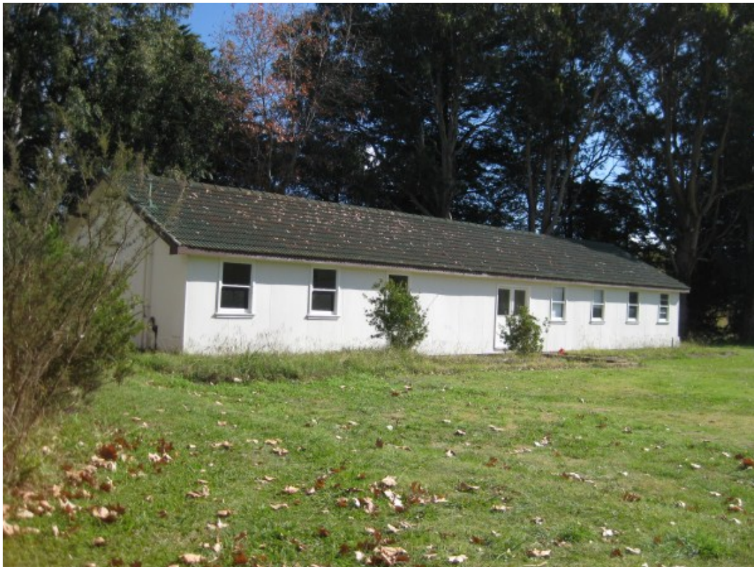
Figure 7.0 Part of the old Reid House Hostel moved to the site in 1973. (Source GML 2012)
