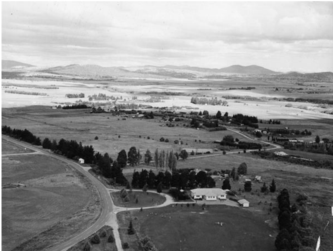
Figure 4.0 Aerial view March 1953 looking southwest over Pialligo. The 1936 school and shelter shed are visible on the site adjacent to the school oval and accessed by a circular entrance drive. What may be the two original toilet blocks are situated to the rear of the school at either side. (Source: ACT Heritage Library 009616)
