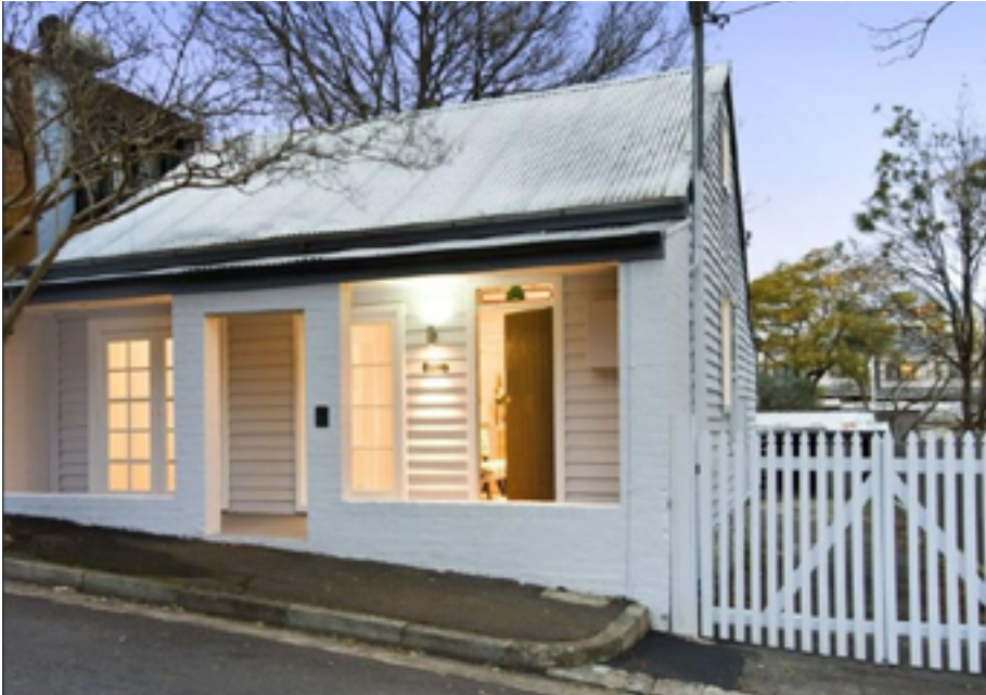
2 Wood Street, Forrest Lodge. The Brüning family home.
