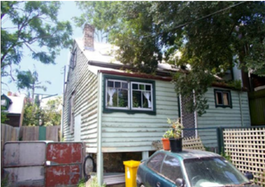
The rear of the house.
