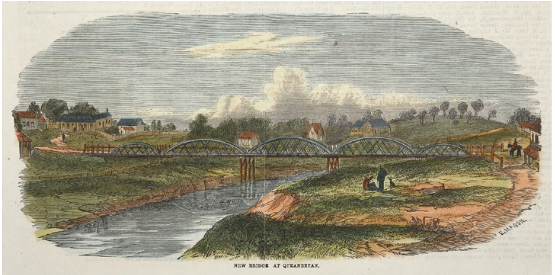
The Queanbeyan Bridge which Joannes helped to repair in 1866.
