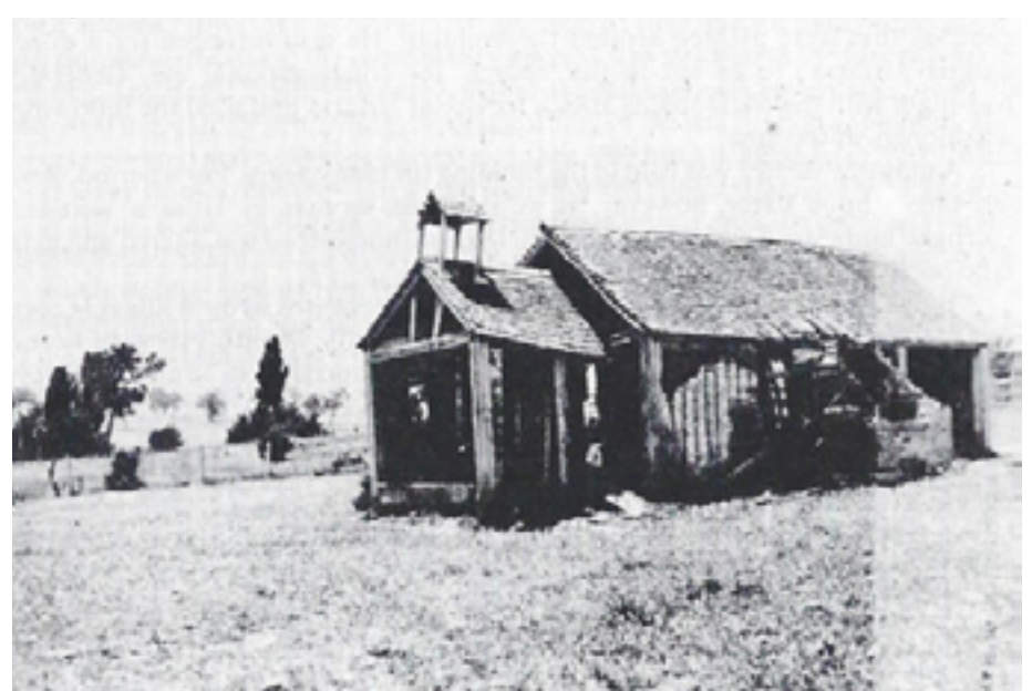
Following its closure in 1902, the building was severely damaged during a storm and allowed to fall into disrepair. Later being used as a stables.
