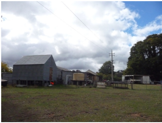
Homestead and outbuilding complex
