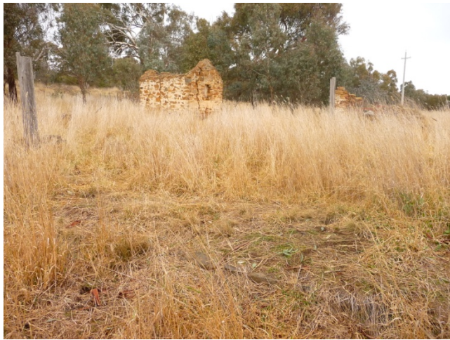
1874 homestead – extent indicated by foundations in foreground, timber beam to LHS and stone ruin to right. A stone outbuilding sits behind the homestead.
